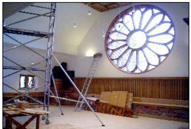
Chester Cathedral's large rehearsal room under construction
