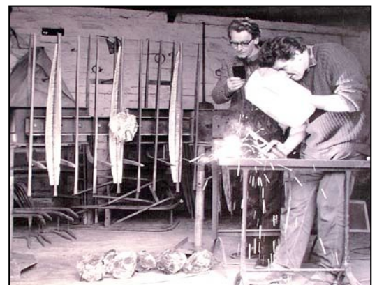
John Hayward watching Tim Reddick constructing the Corona in 1966
